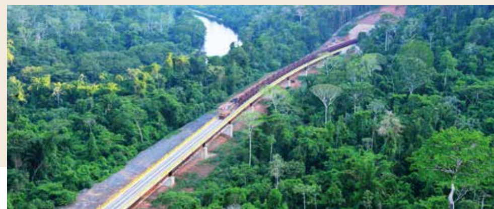
The Vale's SD11 project will allow expanding the Carajás Railroad transportation capacity. Photography: Salviano Machado/Vale Agency
