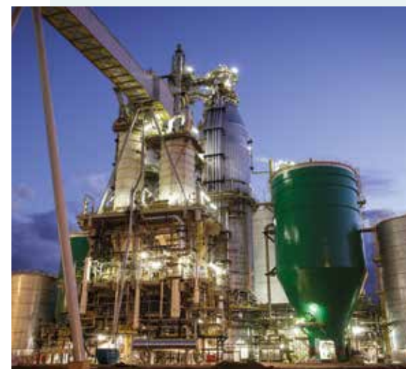
Klabin S.A.'s new pulp mill brings development to the Ortigueira municipality, in Paraná. Photography: Marcio Bruno de Oliveira/Klabin S.A. Collection
